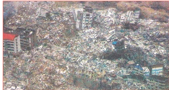
FIGURE 5 Most buildings collapsed in Wenchuan
